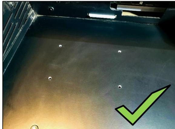
Once the area is clean, lift the console from the front and file out the holes from the underside so they are smooth, and screws will comfortably fit through.
